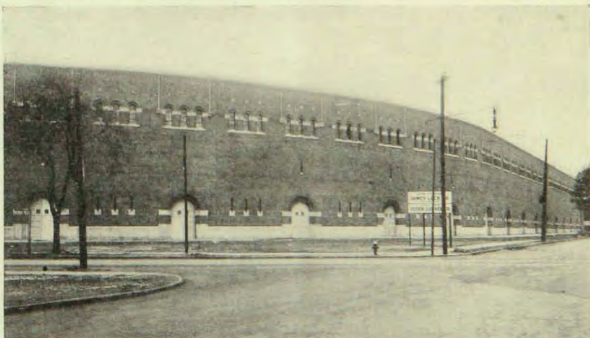
The Memorial Stadium as you approach from St. Paul on University avenue. The curve runs along Oak street, the highway to your left. The graceful dignity of the brick and limestone wall is apparent here. Note the many double entrance doors which lead to the ramps and the flag poles above, included to lend a festive air to the huge amphitheater of sport.
