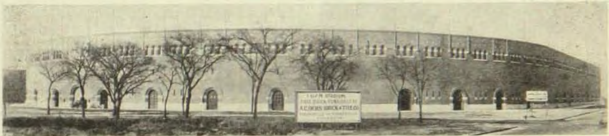
The Memorial Stadium of the University of Minnesota was completed fully 30 days ahead of schedule due to the efficiency of the contractors and the prompt delivery of face brick and tile by the A. C. Ochs Brick and Tile Company. Minneapolis office, 204 South Ninth Street.
