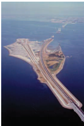
Figure 4.3: Great Belt Crossing – Photograph
