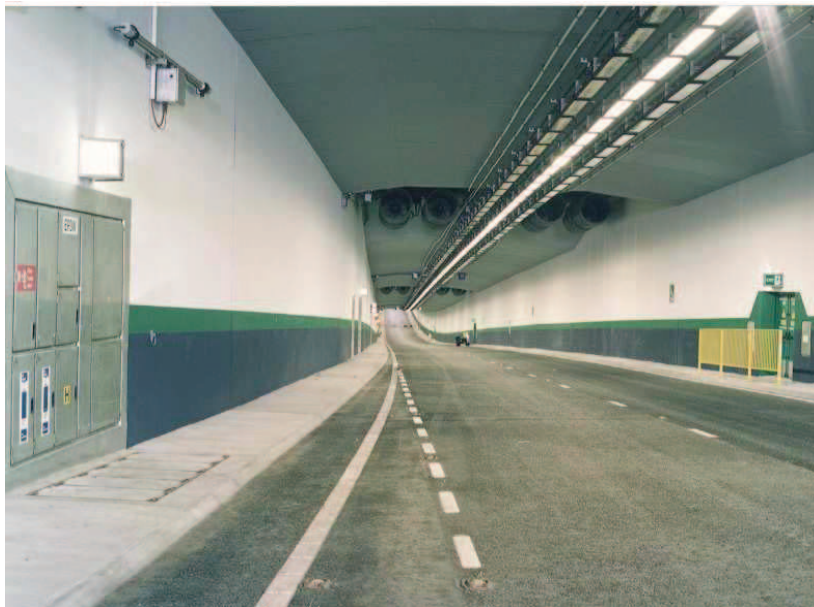
Figure 4.20: Interior of Immersed Tube Tunnel
