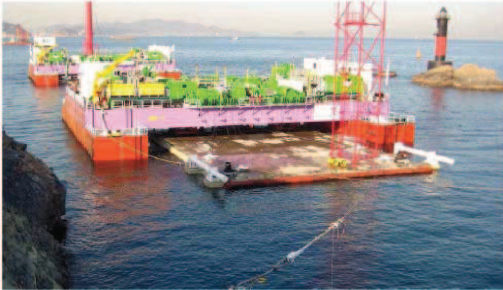
Figure 4.2: Busan Geoje ITT – Floating Out
